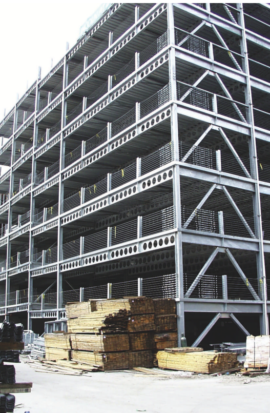
The Delaney Square parking structure in Orlando, Fla. features a galvanized steel frame.
